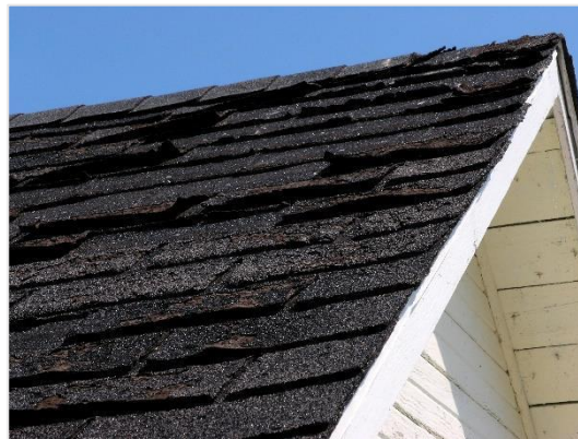
Loose/Brittle Shingles
